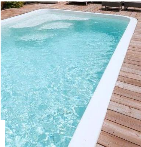
EXPOSED EDGE OF THE POOL
