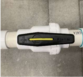
Handle in the direction of the piping = opened valve
