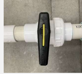
Handle in the opposite direction of the piping = closed valve
